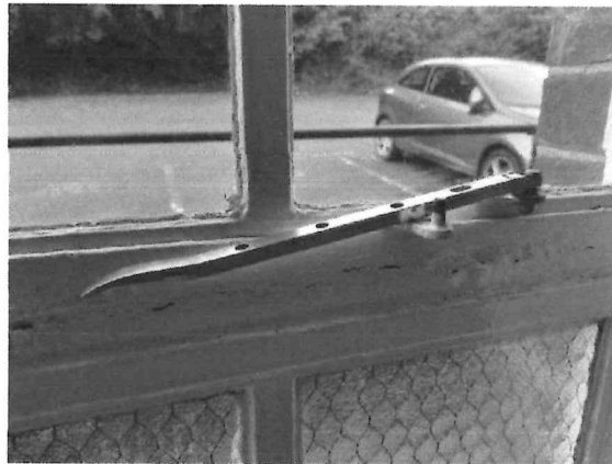
Image 4 Modern window stay does not fit & should be replaced to its original design
