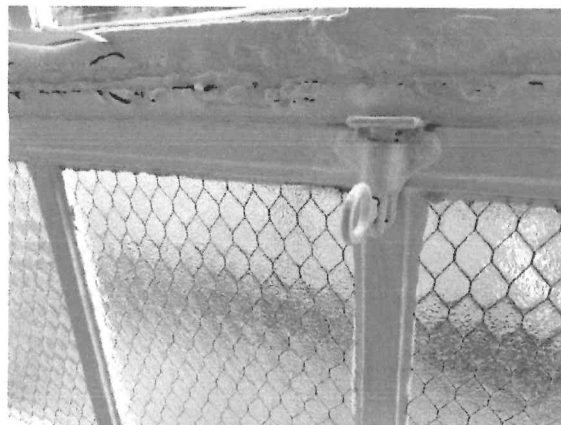
Image 4 Modern window stay does not fit & should be replaced to its original design
