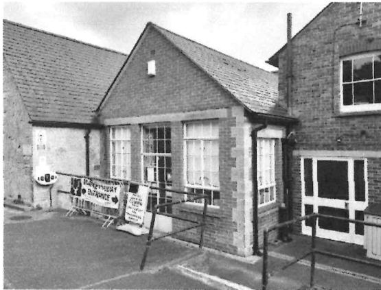
Image 2 Pitched roof extension likely to date from similar period, again with Crittal windows to front & side
