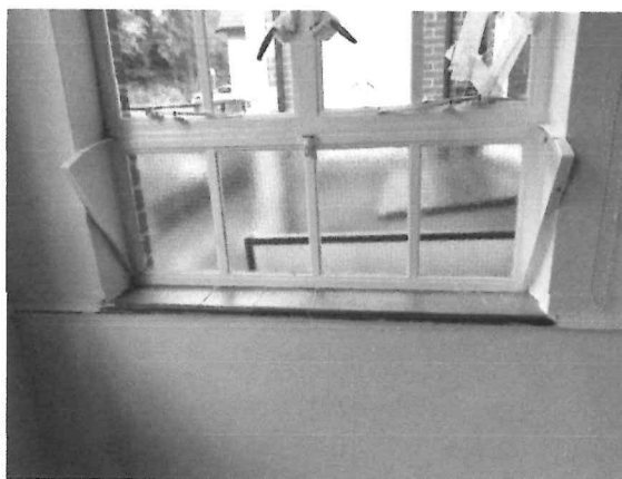
Image 7 Careful design for secondary glazing around fixed bottom casement stays will be required
