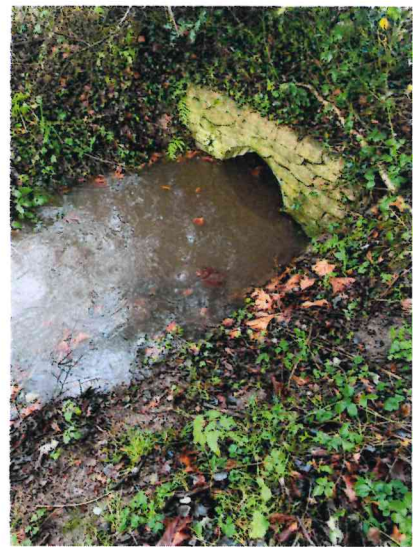
Rush Green exit culvert
