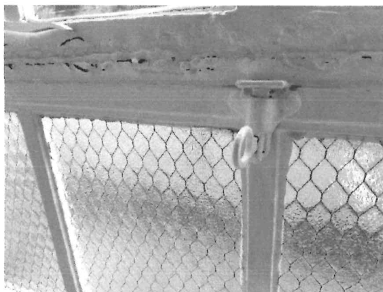
Image 4 Modern window stay does not fit & should be replaced to its original design
