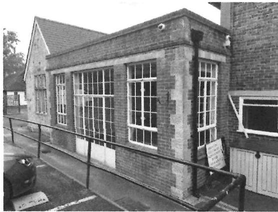
Image 1 Flat roofed 1930's extension with Crittall windows to front & side
