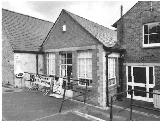
Image 2 Pitched roof extension likely to date from similar period, again with Crittall windows to front & side
